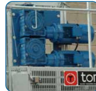
Grupo motriz: motorreductores con electrofreno integrado Drive unit: gearmotors with built-in electric brake
