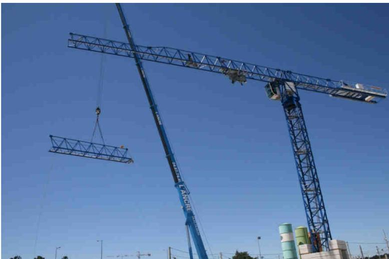
In LINDEN COMANSA flat top tower cranes, a smaller mobile crane is required due to the lower weight of the single jib sections, as opposed to a complete jib. Furthermore the erection of the jib sections is very simple, because the upper part of the union between two jib sections is normally
