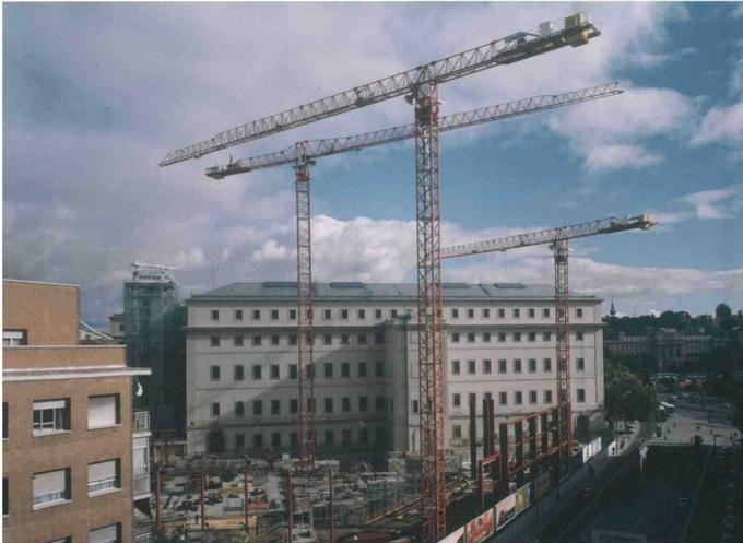
The most typical is very clear: if there is a project in which there will be several cranes working at the same time, and some of them are going to work over between them, working with flat top cranes could give the project manager some definitive advantages by reducing the height between the cranes.
